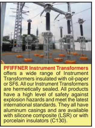
**PFIFFNER** Instrument Transformers offers a wide range of Instrument Transformers insulated with oil-paper or SF6. All our Instrument Transformers are hermetically sealed. All products have a high level of safety against explosion hazards and meet the latest international standards. They all have aluminum casings and are available with silicone composite (LSR) or with porcelain insulators (C130).
